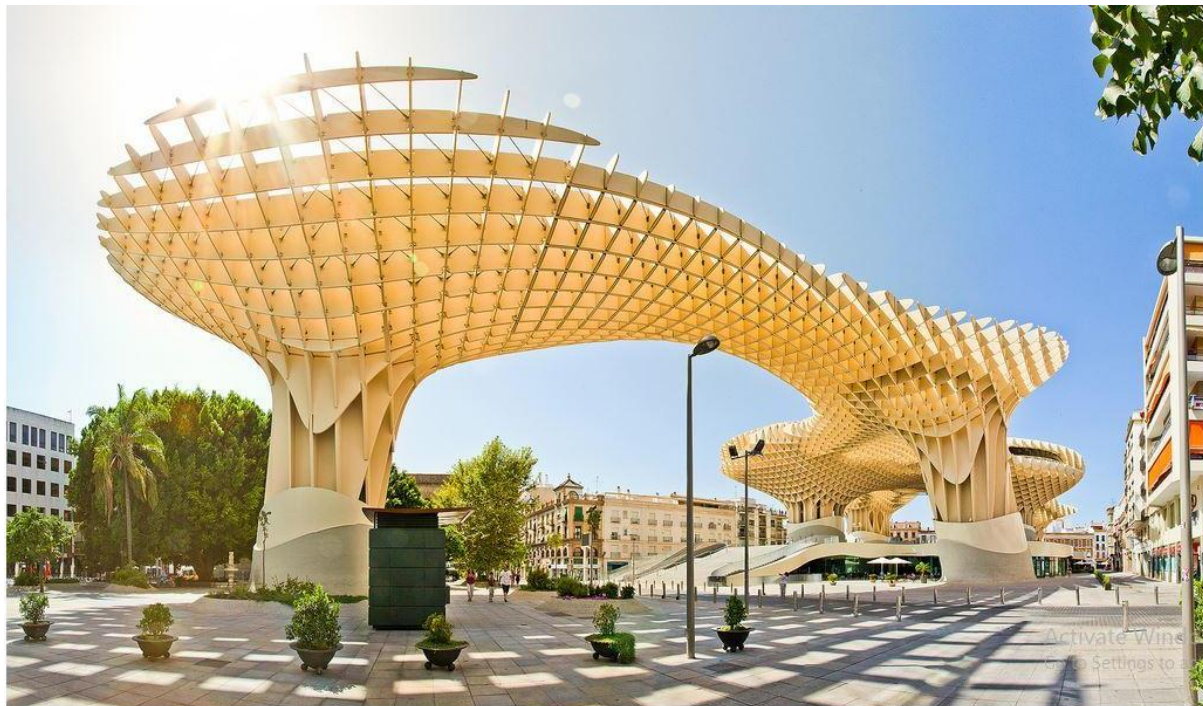
Fig. 15: The “Metropol Parasol” in Seville, the world’s largest wooden structure. Image credit - Inhabitat.
