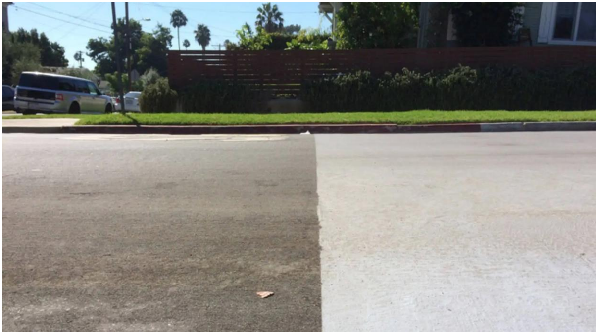
Fig. 13: A stretch of Coronado St. in Los Angeles is one of 15 blocks that is piloting a cool pavement. Image credit - Jed Kim/Marketplace.
